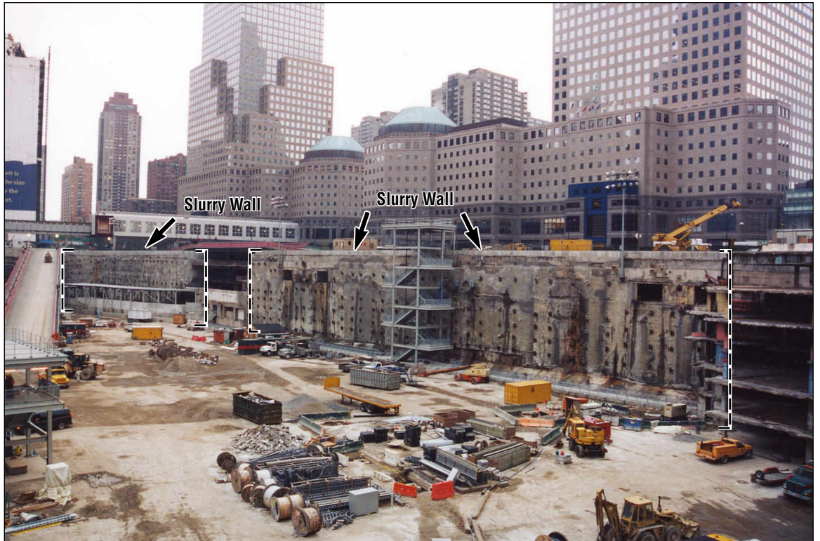
West slurry wall 1
